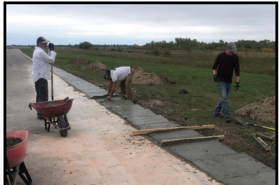
Steve Leiding helps Jim & Chris work the concrete into shape and trowel and broom finish it to a quality finish with 50mm ripples
