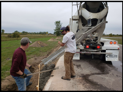
Jim Worton and Chris Gauthier pouring the concrete. A total of 5 yards of high strength concrete was utilized for the new turn 5 exit kerb
