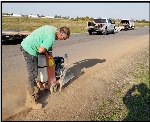
Tom Dwyer working the concrete saw. It's a big job to cut a nice clean edge of the track for the new kerb to butt up against.
