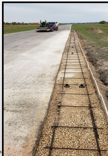
Steve Leiding helps Jim & Chris work the concrete into shape and trowel and broom finish it to a quality finish with 50mm ripples
